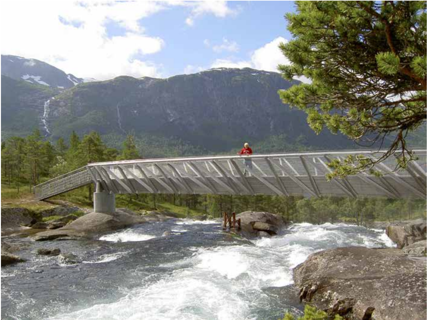
First walkwaybridge in LDX 2101® crossing Likholefossen at Gaularfjell in Norway.
